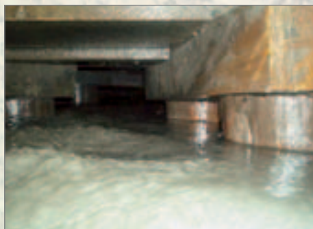
Houten paalfundering in Amsterdam
